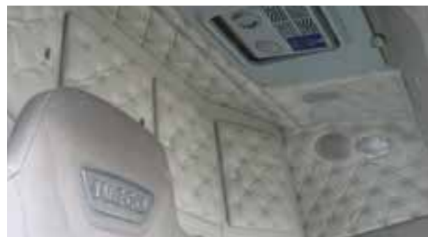
☑ Slight decolouration due to sun rays
