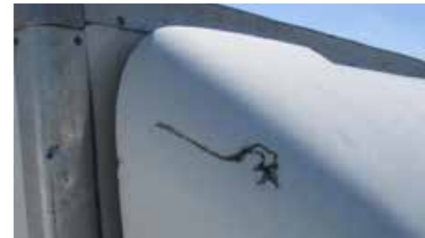
Cabover and deflector: Within economic repair
