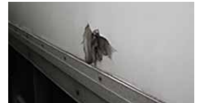
Wood side panels: Damaged wood support greater than 20 cm in length
