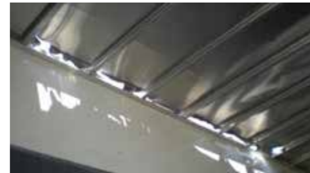
↻ Roof space: Frame damaged, materials not within economic repair
